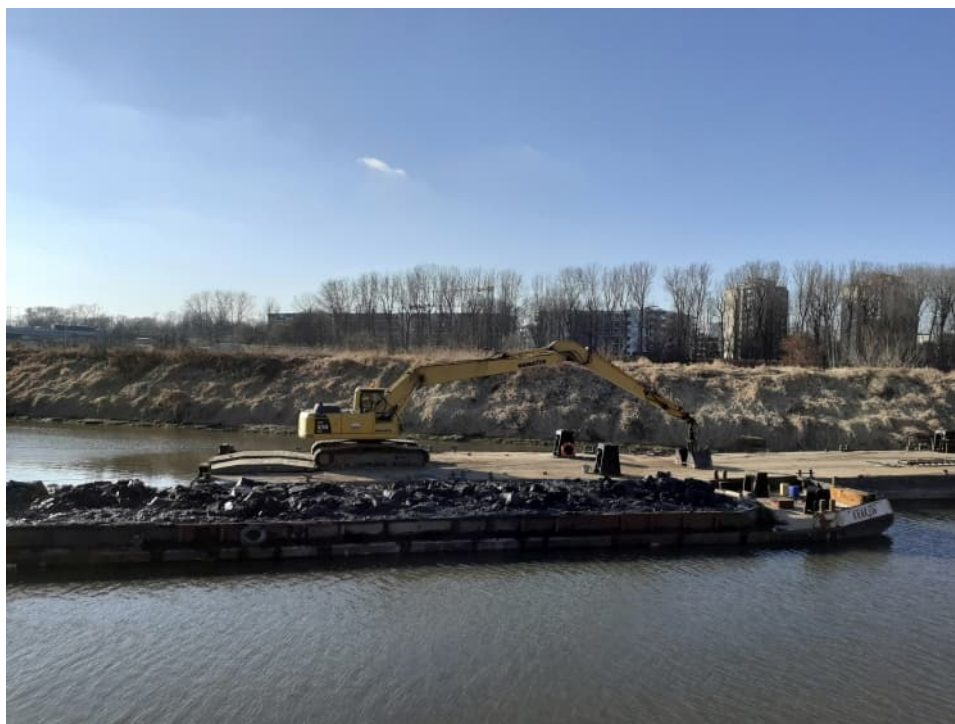
Fig. 33. Dredging of the Płaszów port channel bed north of the flood gate, status in the first decade of March 2022 (view towards the west).
