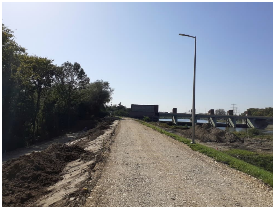
Fig. 55. Covering slopes of the Vistula flood embankment with a top-soil layer, status in the third decade of September 2023 (view towards the west).
