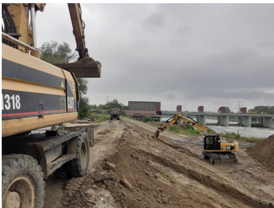
Fig. 53. Shaping slopes of the Vistula flood embankment upstream of the Płaszów port, status in the third decade of August 2023 (view towards the west).
