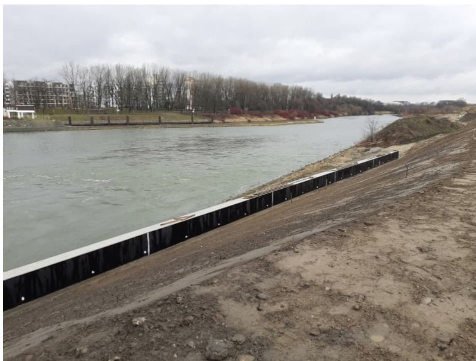
Fig. 54. Shaping slopes of the Vistula flood embankment upstream of the Płaszów port, status in the first decade of March 2023 (view towards the east).
