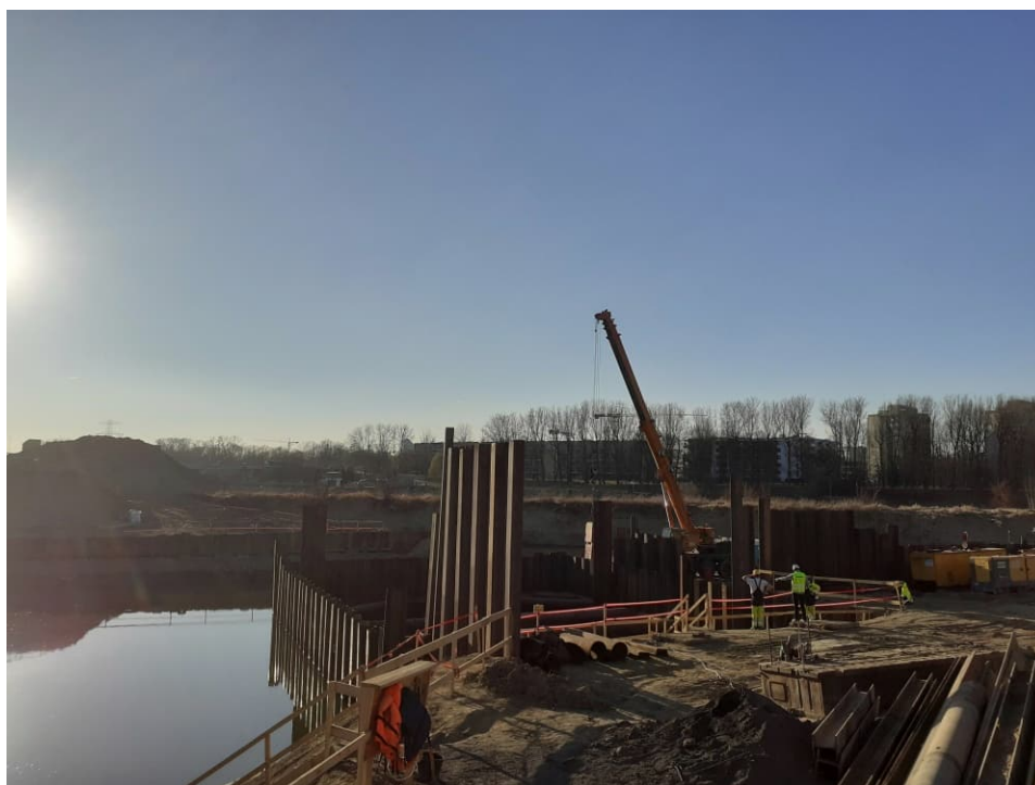
Fig. 36. Driving the sheet piles on the eastern bank of the Płaszów port channel, status in the third decade of March 2022 (view towards the west).
