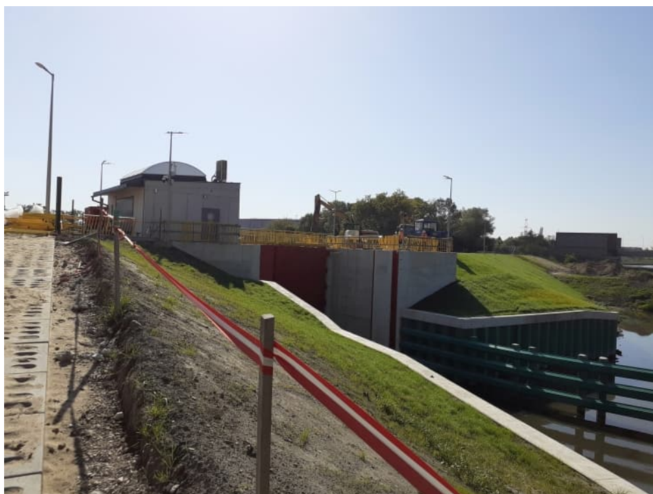
Fig. 58. Growth of grasses sown on the slopes of the Vistula flood embankment and on the bank slope of the Płaszów port channel, status in the third decade of September 2023 (view towards the west).
