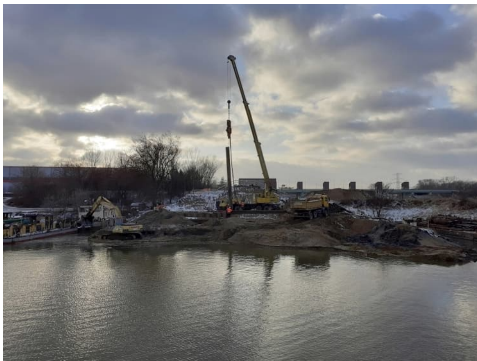
Fig. 35. Driving the sheet piles on the western bank of the Płaszów port channel, status in the second decade of January 2022 (view towards the west).
