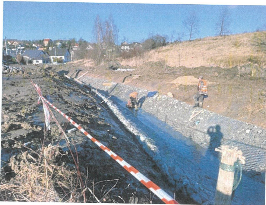
Fig. 55. Reinforcements of the Malinówka stream bed in the upstream part of reservoir, status in the third decade of January 2025 (view towards the west).
