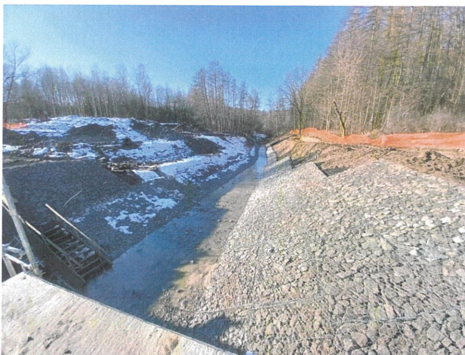
Fig. 53. Reinforcements of the Malinówka stream bed downstream of the reservoir's spillway-discharge facilities, status in the third decade of January 2025 (view towards the west).
