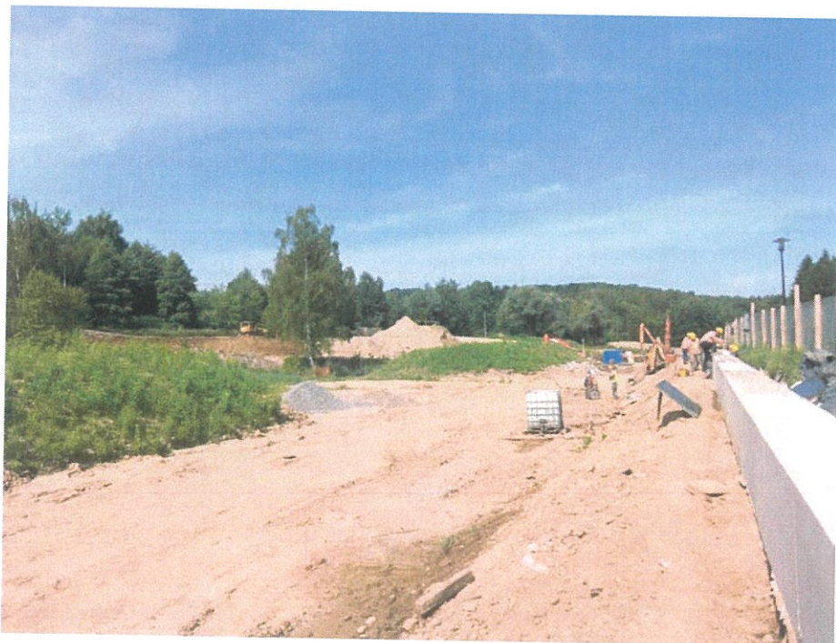
Fig. 32. Making a cap on the sheet pile wall along the northern bank of the reservoir, status in the third decade of June 2024 (view towards the west).
