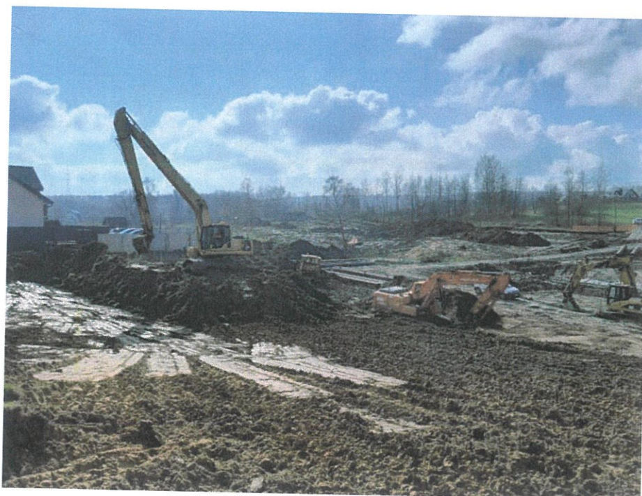
Fig. 24. Removal of a top soil layer on the northern bank of reservoir, status in the second decade of March 2024 (view towards the east).
