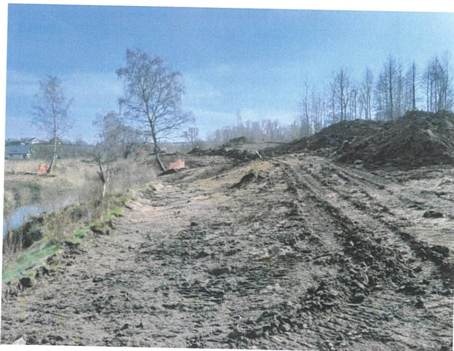
Fig. 23. Removal of a top soil layer on the southern bank of reservoir, status in the second decade of March 2024 (view towards the east).
