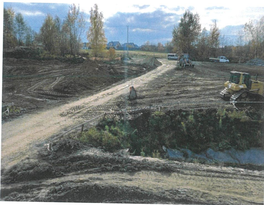
Fig. 60. Covering the reservoir bowl on the southern bank of the Malinówka stream with a top-soil layer, status in the third decade of October 2024 (view towards the south).
