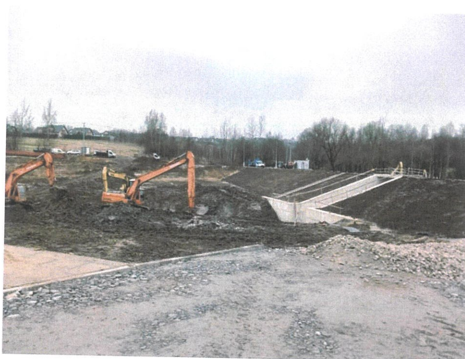
Fig. 44. Construction site of the front dam and the reservoir's spillway-discharge facilities, status in the first decade of April 2025 (view from the northern bank of the reservoir, towards the south).
