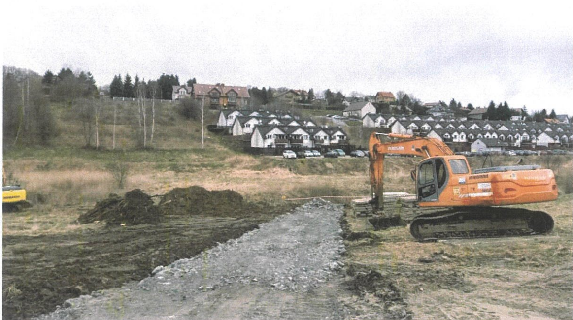
Fig. 13. Construction of a technological road to the building place of reservoir's front dam, status in the third decade of February 2024 (view towards the north).
