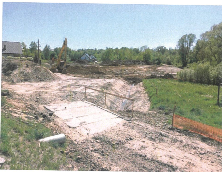
Fig. 51. Reconstruction of the R4 ditch in the northern part of the reservoir basin, status in the third decade of April 2024 (view towards the south-east).
