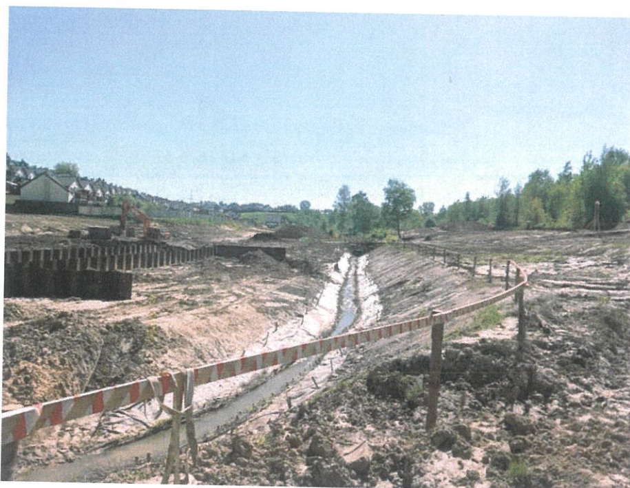
Fig. 28. Malinówka stream bypass channel for the period of construction of the reservoir dam, status in the third decade of April 2024 (view towards the west).
