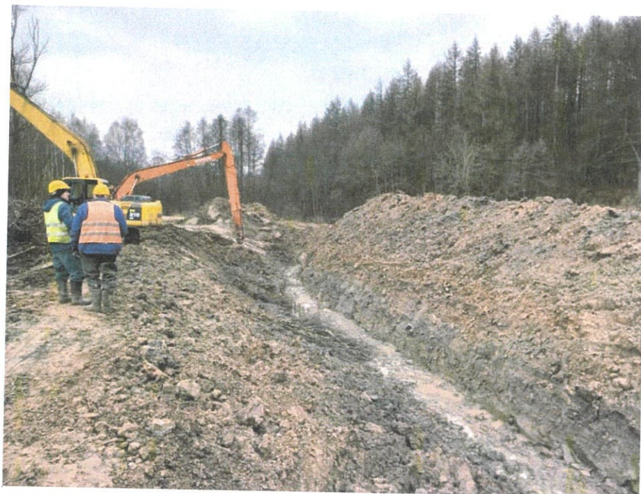
Fig. 27. Construction of the Malinówka stream bypass channel for the period of construction of the reservoir dam, status in the third decade of February 2024 (view towards the west).
