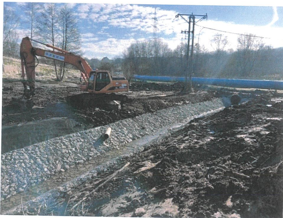
Fig. 56. Reinforcements of the Malinówka stream bed in the upstream part of reservoir, status in the first decade of February 2025 (view towards the east).
