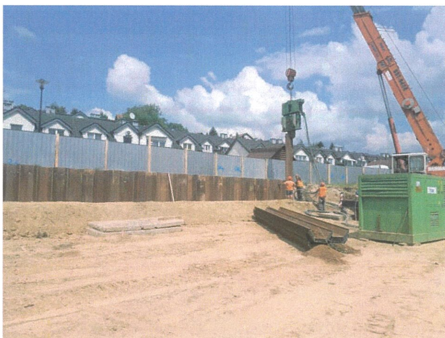
Fig. 30. Driving the sheet piles along the northern bank of the reservoir, status in the third decade of May 2024 (view towards the north).
