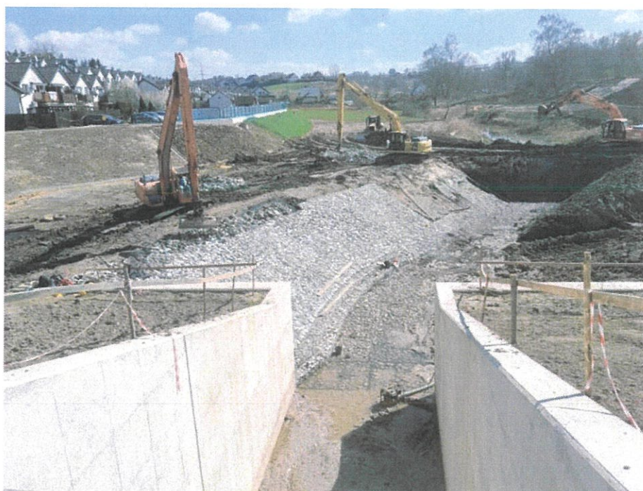
Fig. 54. Reinforcements of the Malinówka stream bed upstream of the reservoir's spillway-discharge facilities, status in the first decade of April 2025 (view towards the east).
