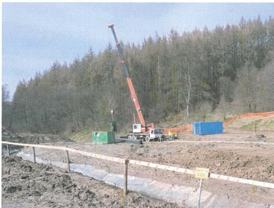
Fig. 29. Driving the sheet piles on the construction site of the reservoir's front dam, status in the second decade of March 2024 (view towards the west).
