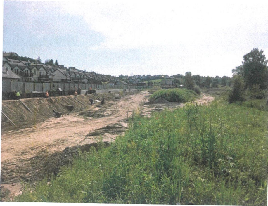
Fig. 31. Making a cap on the sheet pile wall along the northern bank of the reservoir, status in the third decade of June 2024 (view towards the east).
