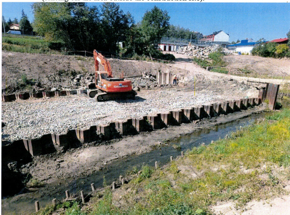
Foto. 8. Serafa 2 reservoir , third decade of July 2022 (construction of a discharge and overflow device, fence in the background).
