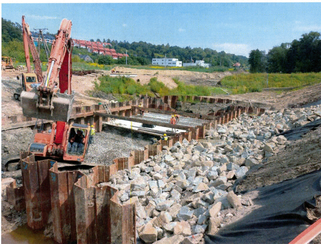
Foto. 10. Serafa 2 reservoir , second decade of August 2022 (construction of a discharge and overflow device).
