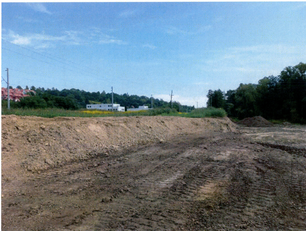
Foto. 9. Serafa 2 reservoir , first decade of August 2022 (forming the reservoir embankment and shaping the reservoir bowl).
