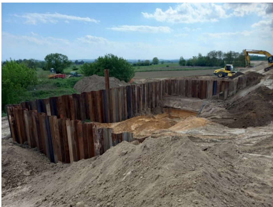
Fig. 35. Reconstruction of the embankment culvert – the left Vistula embankment within Section 2 , status in the second decade of May 2022 (view towards the embanked area).
