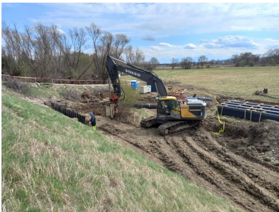
Fig. 33. Construction of a sheet piling barrier along the base of embankment – the left Vistula embankment within Section 1.1 , status in the first decade of April 2022 (downstream view).
