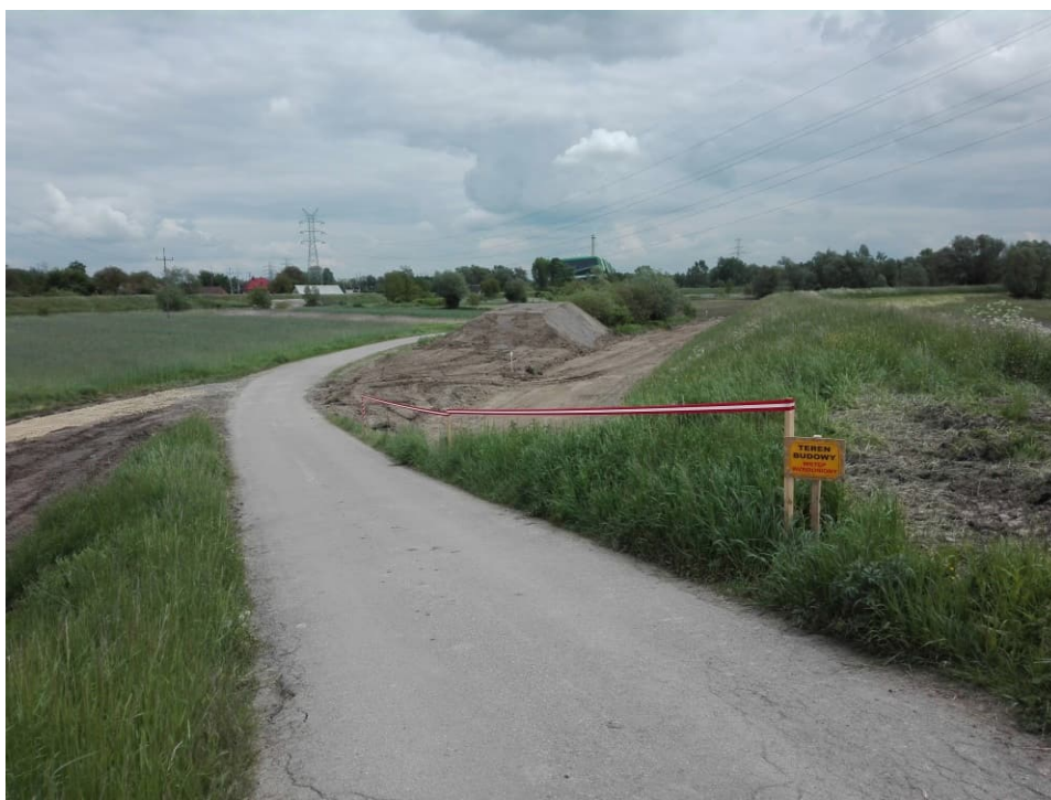
Fig. 29. Protection of top-soil piles – the right Dłubnia embankment within Section 1.4 , status in the third decade of May 2022 (downstream view).
