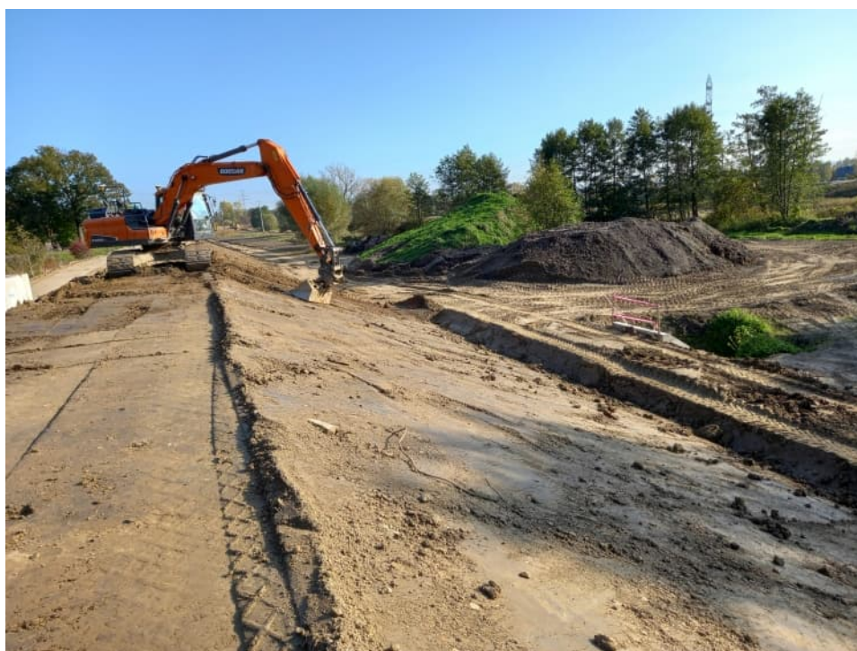
Fig. 42. Leveling the slopes of the flood embankment – the left Dłubnia embankment within Section 1.6 , status in the second decade of October 2022 (downstream view).
