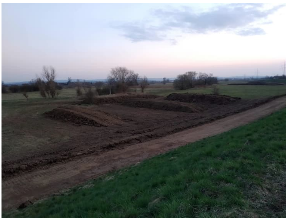
Fig. 30. Protection of top-soil piles – the left Vistula embankment within Section 2 , status in the third decade of July 2021 (upstream view).
