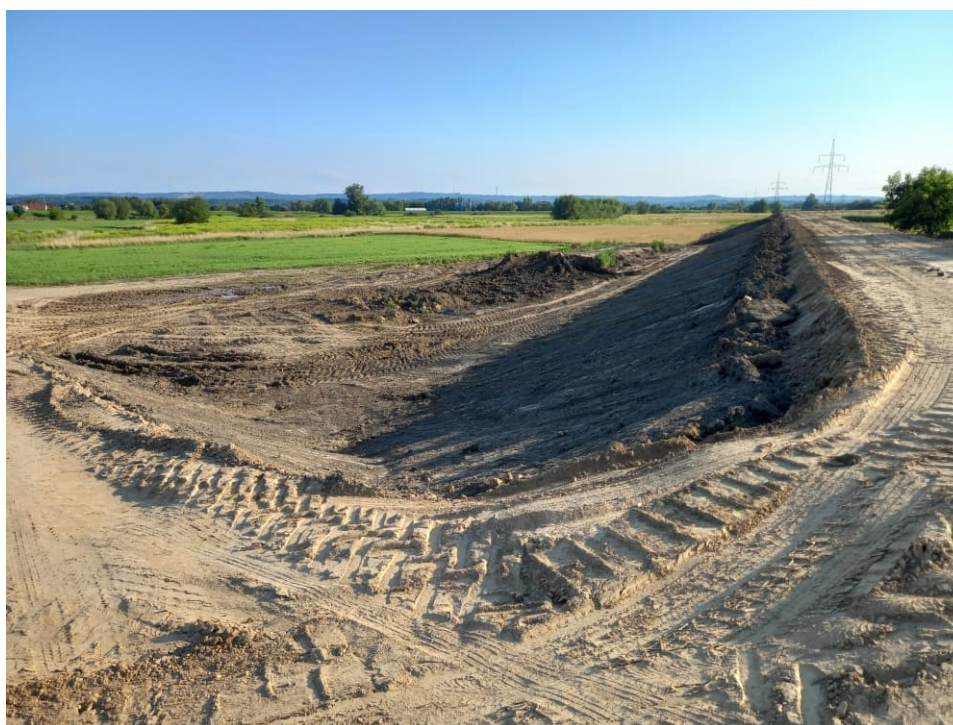
Fig. 46. Covering slopes of the flood embankment with a top-soil layer – the left Vistula embankment within Section 2 , status in the third decade of July 2022 (upstream view).
