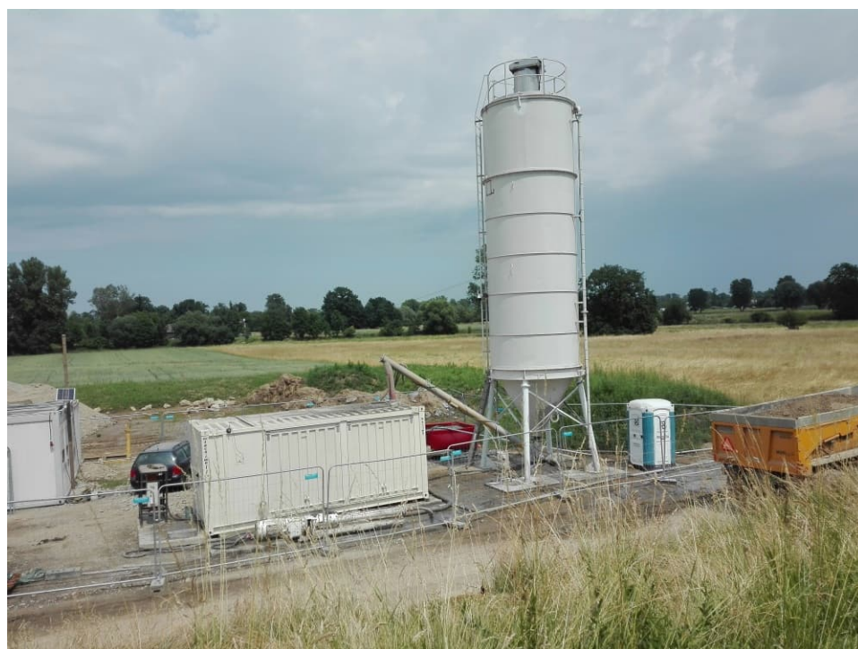
Fig. 32. Installation for producing a cement-bentonite mixture – the left Vistula embankment within Section 2 , status in the third decade of June 2021 (downstream view).
