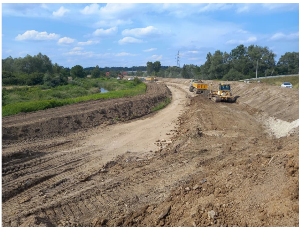
Fig. 40. Shaping the slopes of the flood embankment – the left Dłubnia embankment within Section 1.5 , status in the third decade of July 2022 (upstream view).
