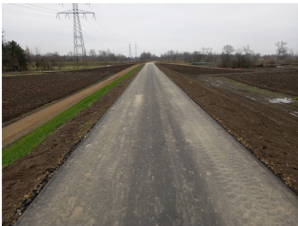
Fig. 48. Construction of a road on the crown of the flood embankment – the left Vistula embankment within Section 2 , status in the third decade of November 2022 (downstream view).
