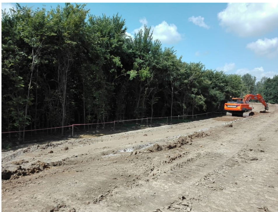
Fig. 21. Protection of trees and shrubs not intended to felling – the left Vistula embankment within Section 1.3 , status in the second decade of August 2022 (upstream view).
