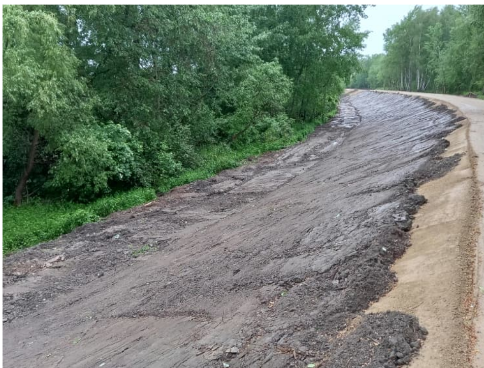
Fig. 45. Covering slopes of the flood embankment with a top-soil layer – the left Vistula embankment within Section 1.3 , status in the third decade of May 2022 (upstream view).
