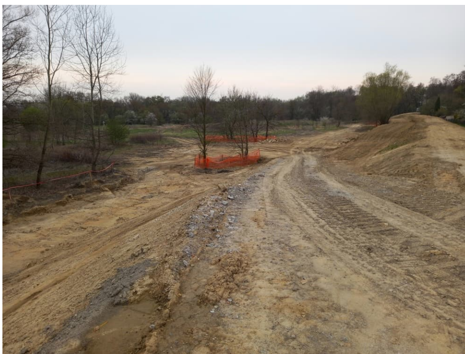
Fig. 22. Protection of trees and shrubs not intended to felling – the left Vistula embankment within Section 2 , status in the second decade of April 2022 (upstream view).
