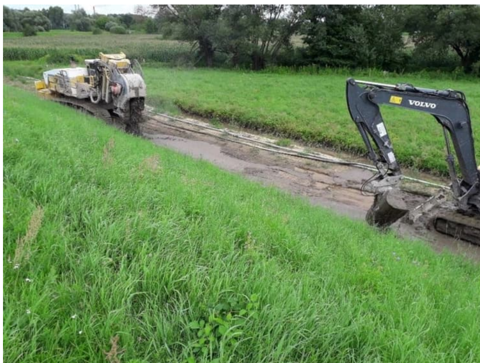
Fig. 31. Construction of a cement-bentonite barrier along the base of embankment – the right Dłubnia embankment within Section 1.4 , status in the second decade of August 2021 (upstream view).
