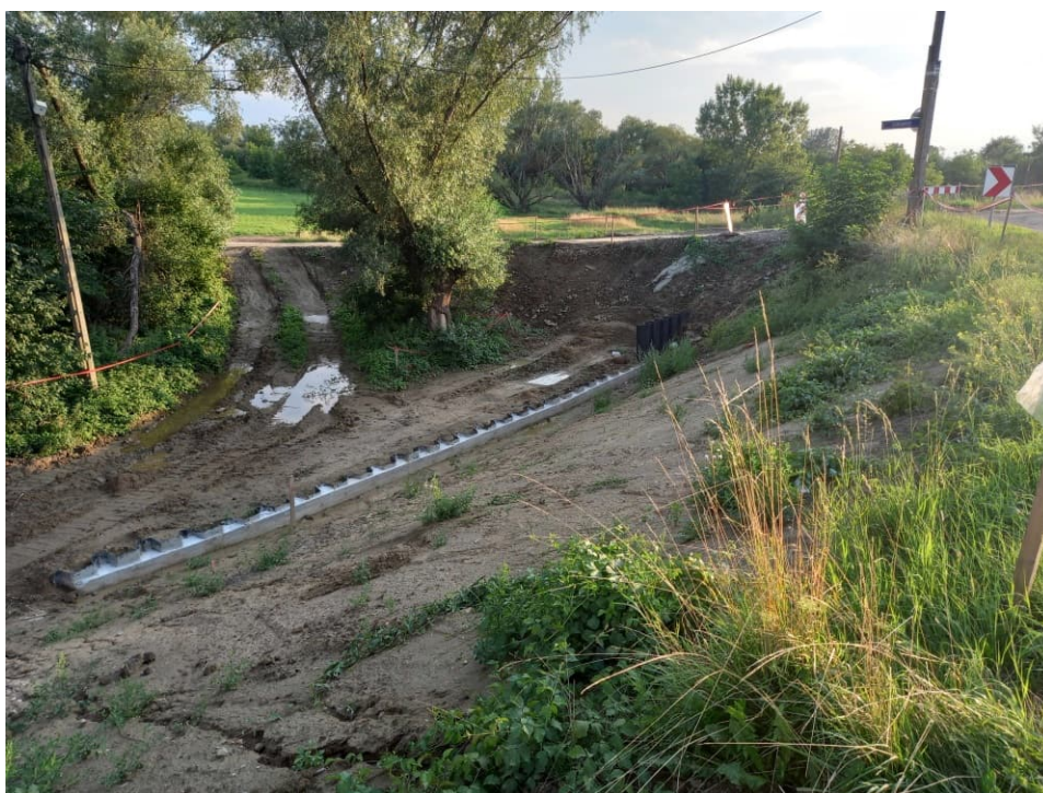
Fig. 34. Making a cap on the sheet pilings along the base of embankment – the left Vistula embankment within Section 1.1 , status in the third decade of July 2022 (upstream view).
