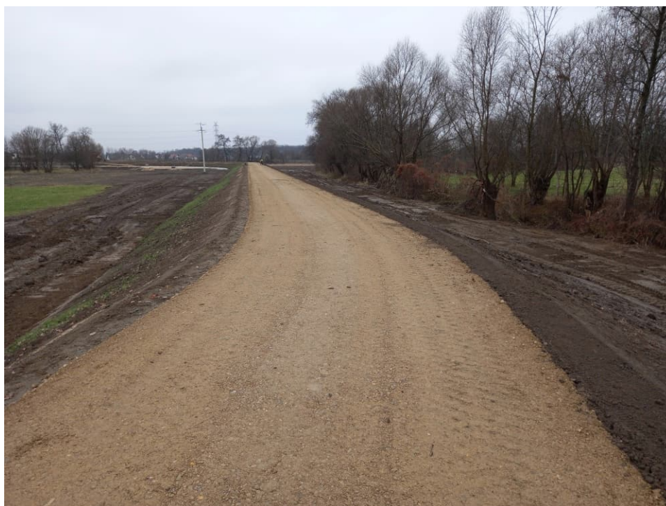
Fig. 47. Construction of a road on the crown of the flood embankment – the left Dłubnia embankment within Section 1.6 , status in the third decade of November 2022 (downstream view).
