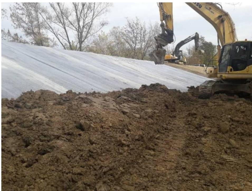
Fig. 43. Placement of bentomat on the slope of the flood embankment – the left Vistula embankment within Section 1.2 , status in the third decade of October 2021 (downstream view).
