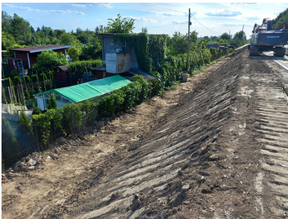
Fig. 41. Leveling the slopes of the flood embankment – the left Vistula embankment within Section 1.1 , status in the second decade of June 2022 (upstream view).
