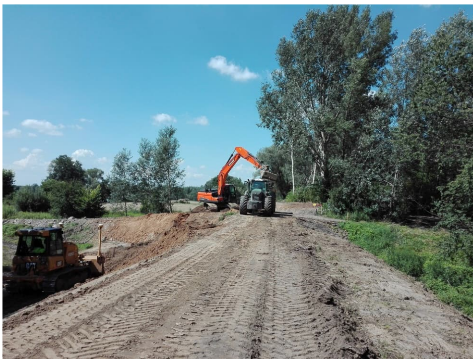
Fig. 27. Removal of a top soil layer – the left Vistula embankment within Section 1.3 , status in the third decade of July 2021 (upstream view).
