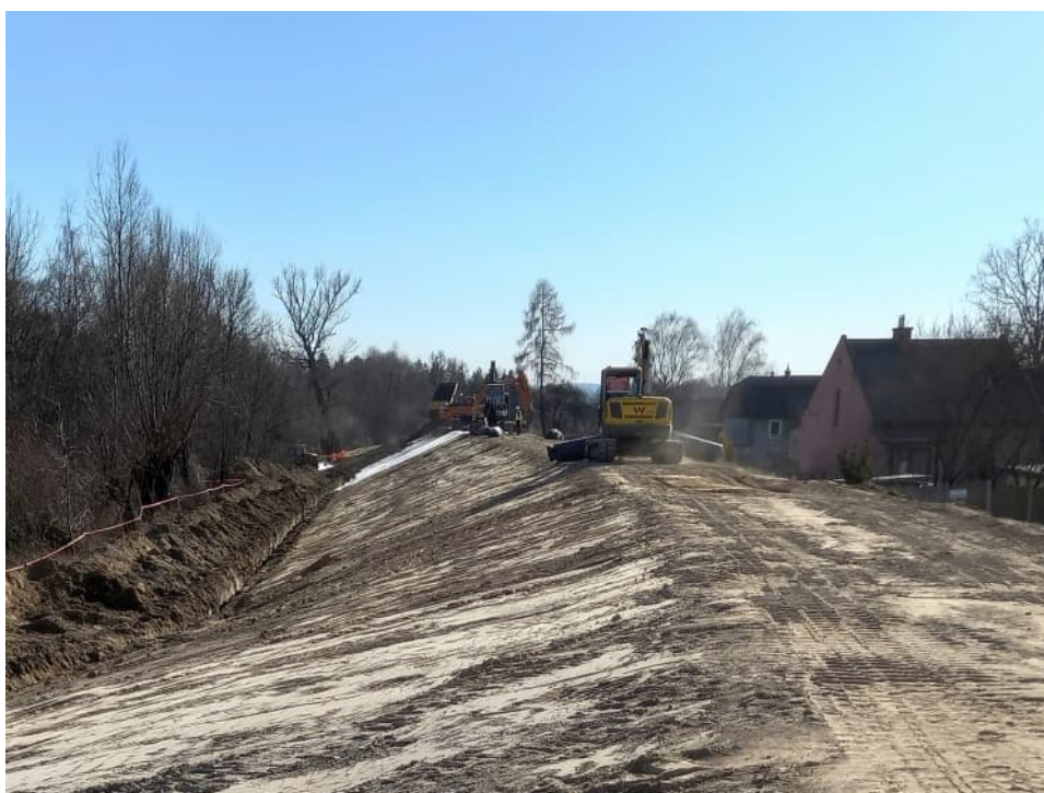
Fig. 44. Placement of bentomat on the slope of the flood embankment – the right Dłubnia embankment within Section 1.4 , status in the third decade of March 2021 (downstream view).
