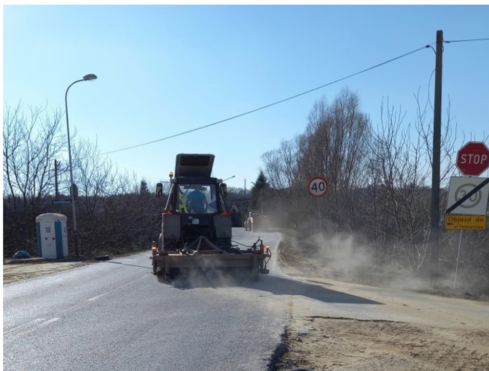
Fig. 25. Keeping public roads clean in the vicinity of the construction site – the right Dłubnia embankment within Section 1.4 , status in the third decade of March 2022 (view towards the west).
