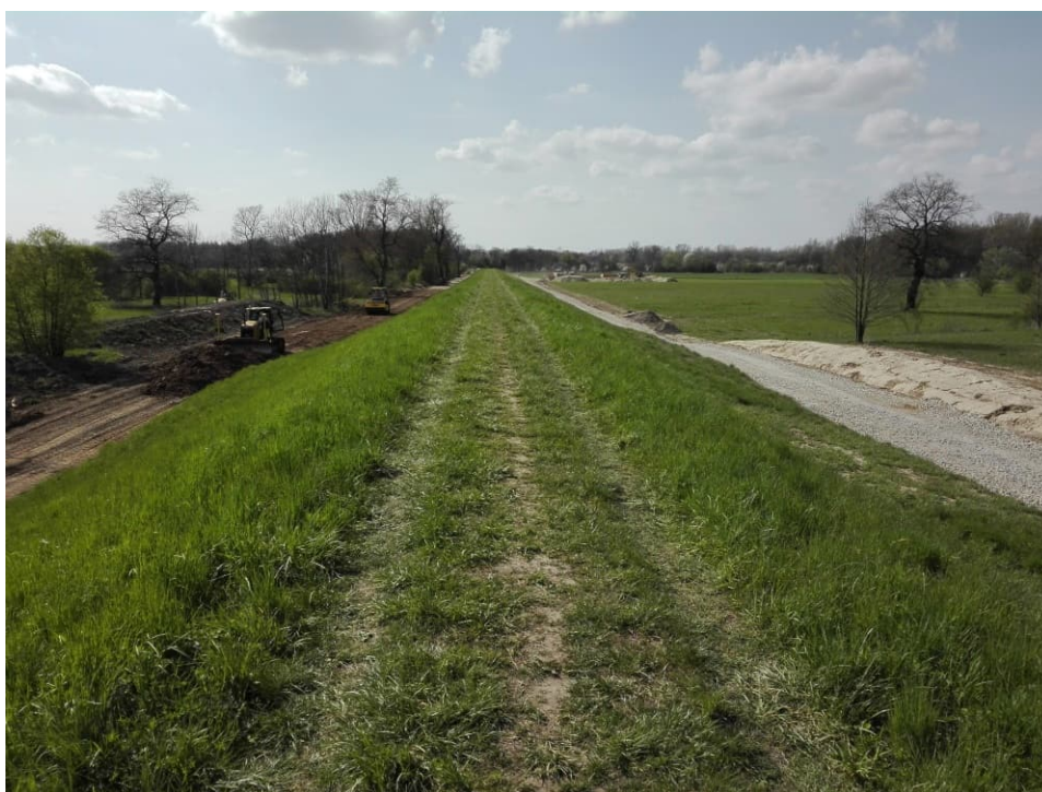
Fig. 28. Removal of a top soil layer – the left Vistula embankment within Section 2 , status in the third decade of July 2021 (upstream view).
