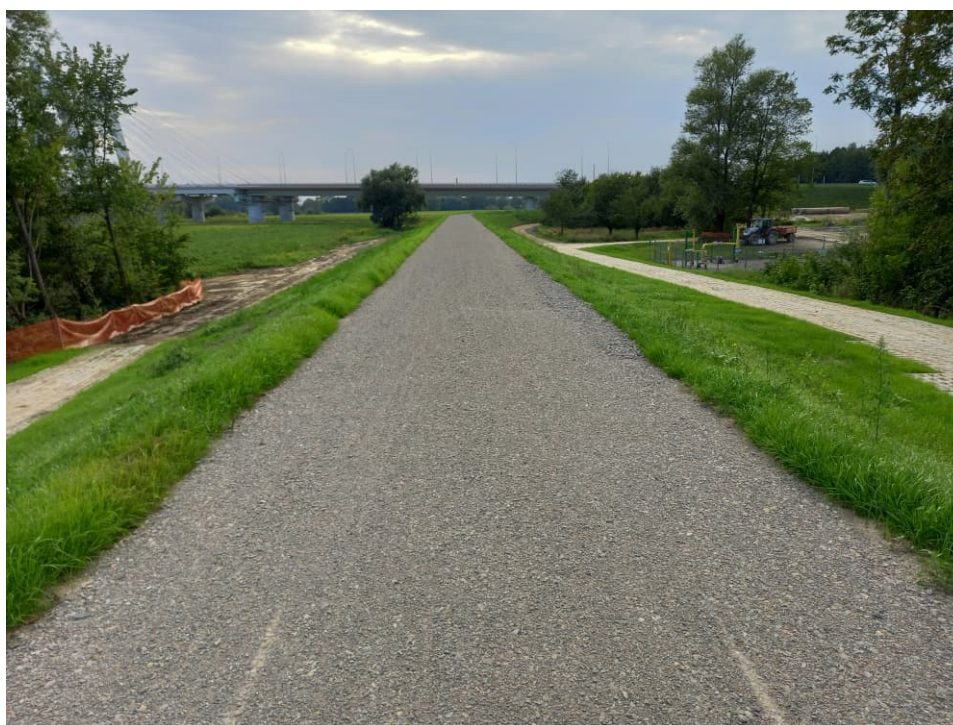
Fig. 50. Growth of grasses sown on the slope of the flood embankment – the left Vistula embankment within Section 1.2 , status in the third decade of August 2022 (upstream view).
