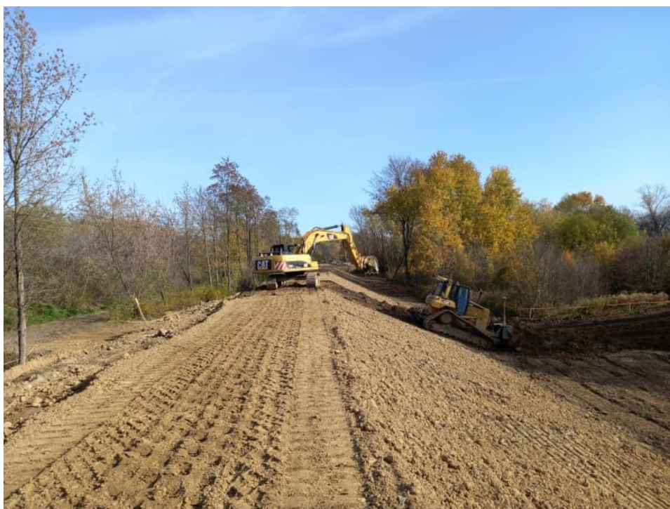
Fig. 39. Shaping the slopes of the flood embankment – the left Vistula embankment within Section 1.2 , status in the third decade of October 2021 (downstream view).
