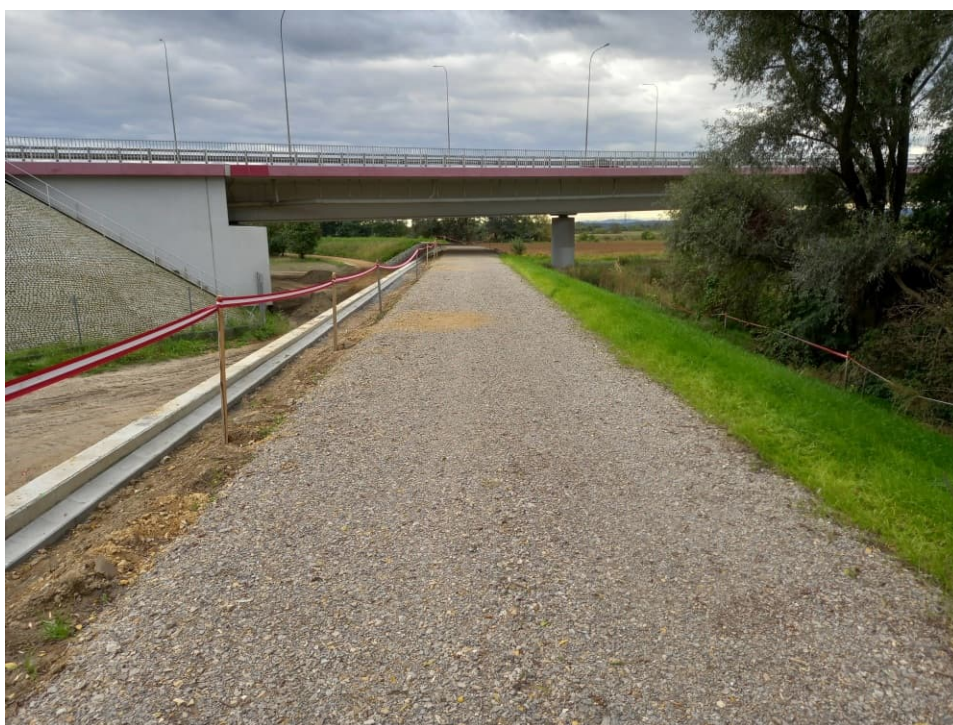
Fig. 18. Protection of hazardous sites – the left Dłubnia embankment within Section 1.5 , status in the third decade of September 2022 (downstream view).
