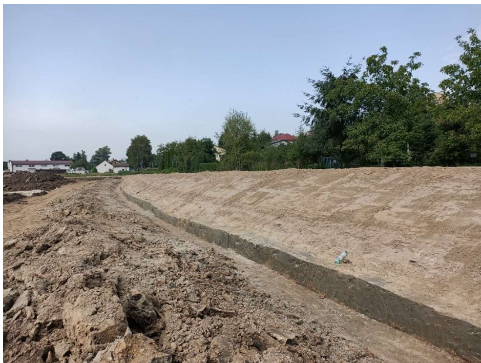
Foto. 9. Malinówka 1 reservoir , third decade of August 2022 (forming the embankment - embanking the reservoir).
