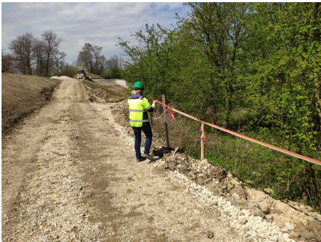
Phot. 17. Left embankment at km approx. 5+200 – reconstruction of damaged greenery fences (2nd decade of April, 2023).
