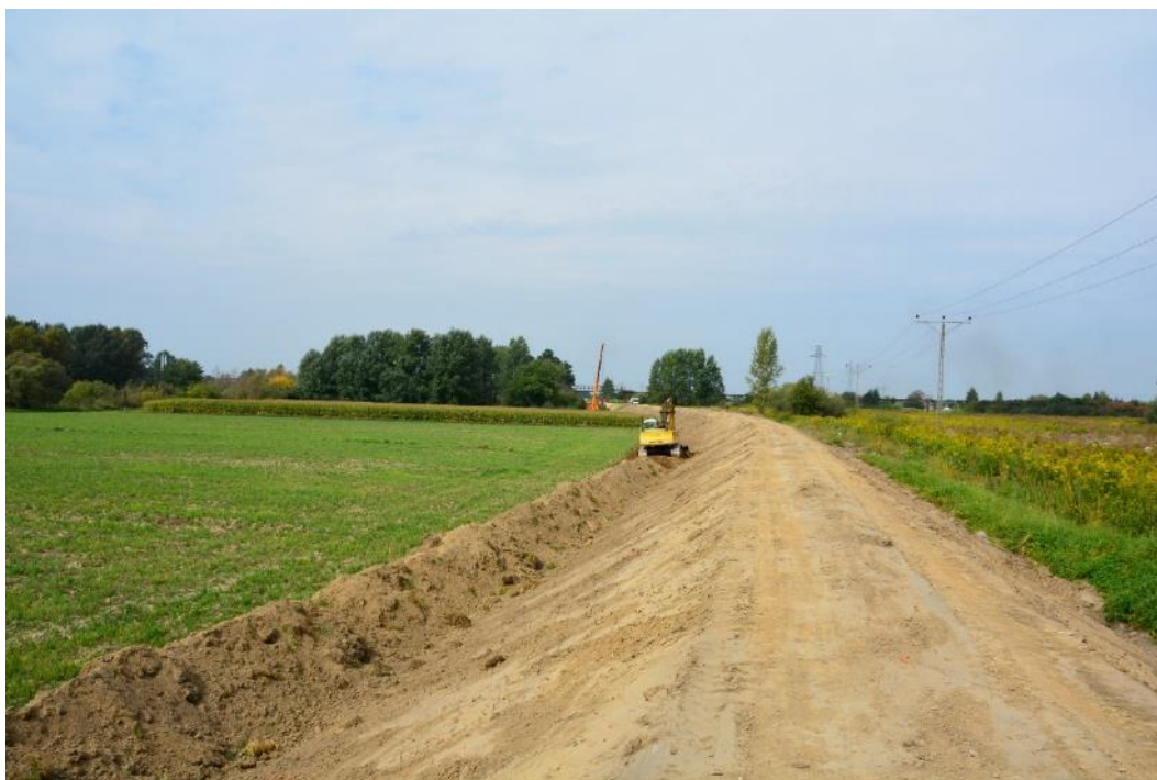
Phot. 2. Right embankment at km approx. 1+200 – topsoil removal of the embankment, maintaining the correct height of topsoil heaps (2nd decade of September, 2021).
