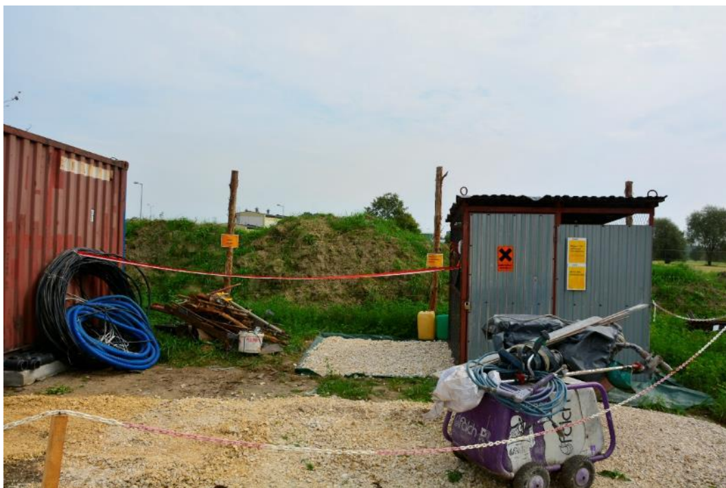
Phot. 6. Control of the Contractor's site facilities zone, view of the prepared area for the storage of hazardous substances and the sorbent access area ("ecological first aid kit") (2nd decade of September, 2021).
