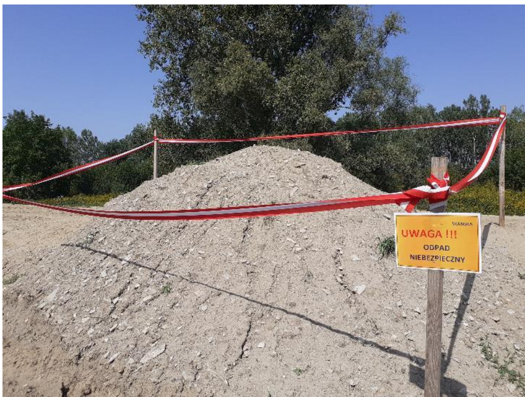
Phot. 11. Left embankment at km approx. 1+100 – example of marking of storage zones for waste discovered during earthworks (soil mixed with asbestos fragments) (3rd decade of August 2022).
