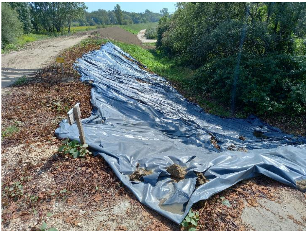
Phot. 12. Right embankment at km approx. 0+900 – example of measures to reduce the growth of invasive plants by covering with plastic sheeting (3rd decade of August 2022).
