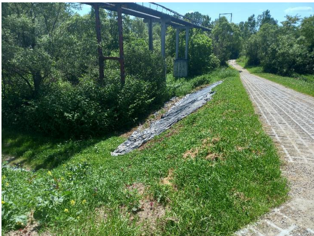
Phot. 18. Right embankment at km approx. 0+500 – measures to reduce the growth of invasive plants (knot weeds) by covering with plastic sheeting (3rd decade of May 2023).
