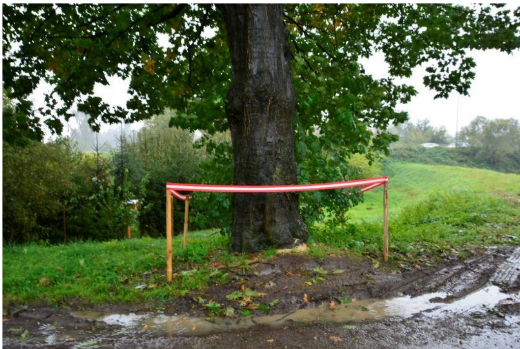
Phot. 7. Right embankment at km approx. 3+200 – example of the constructed greenery fencing (3rd decade of September, 2021).
