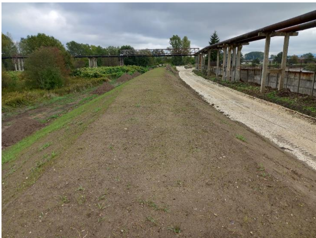
Phot. 14. Left embankment at km approx. 1+200 – example of executing topsoiling and sowing works for the section of the embankment (3rd decade of September, 2022).
