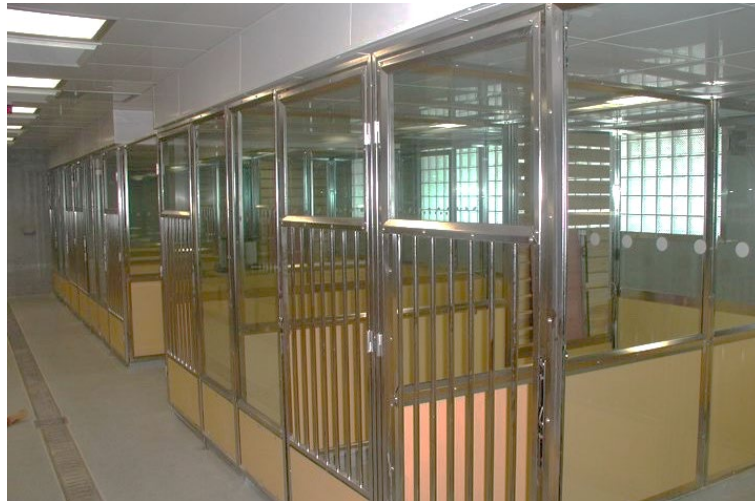
Figure 5.17. Dog unit fitted with glass bricks to let in daylight while maintaining security
