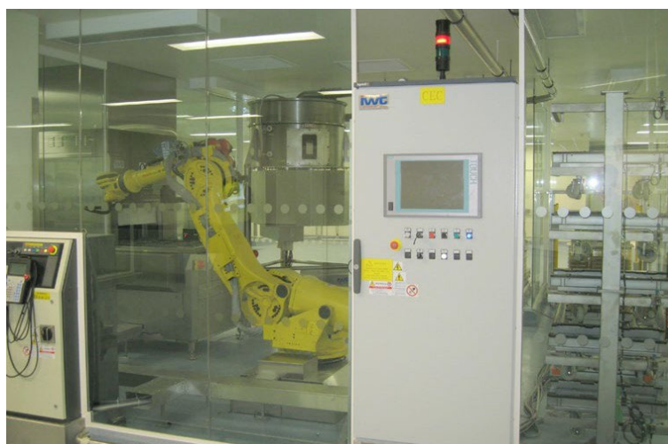
Figure 6.3. Robot working in a cage wash area
