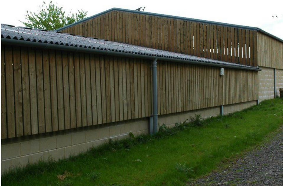
Figure 5.14. Farm animal housing showing a solid wall base topped with weatherboarding. This arrangement allows an adequate airflow above the animals while protecting them from draughts
