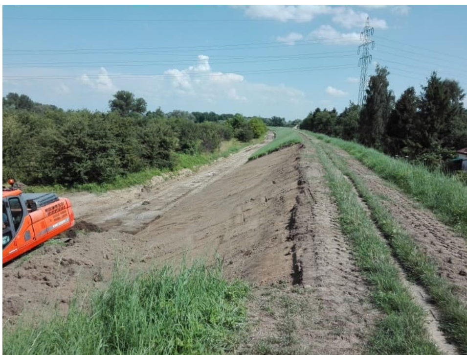
Fig. 30. Removal of a top soil layer – the right Vistula embankment within Section 3.2a , status in the third decade of July 2021 (downstream view).
