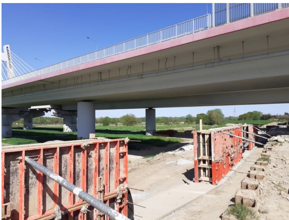
Fig. 40. Construction of a retaining wall – the right Vistula embankment within Section 3.3 , status in the first decade of May 2022 (downstream view).
