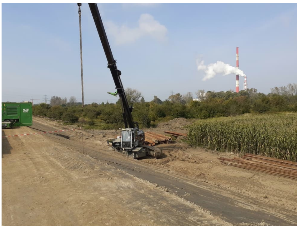
Fig. 35. Construction of a sheet piling to protect the embankment culvert during reconstruction – the right Vistula embankment within Section 3.2a , status in the third decade of September 2021 (upstream view).
