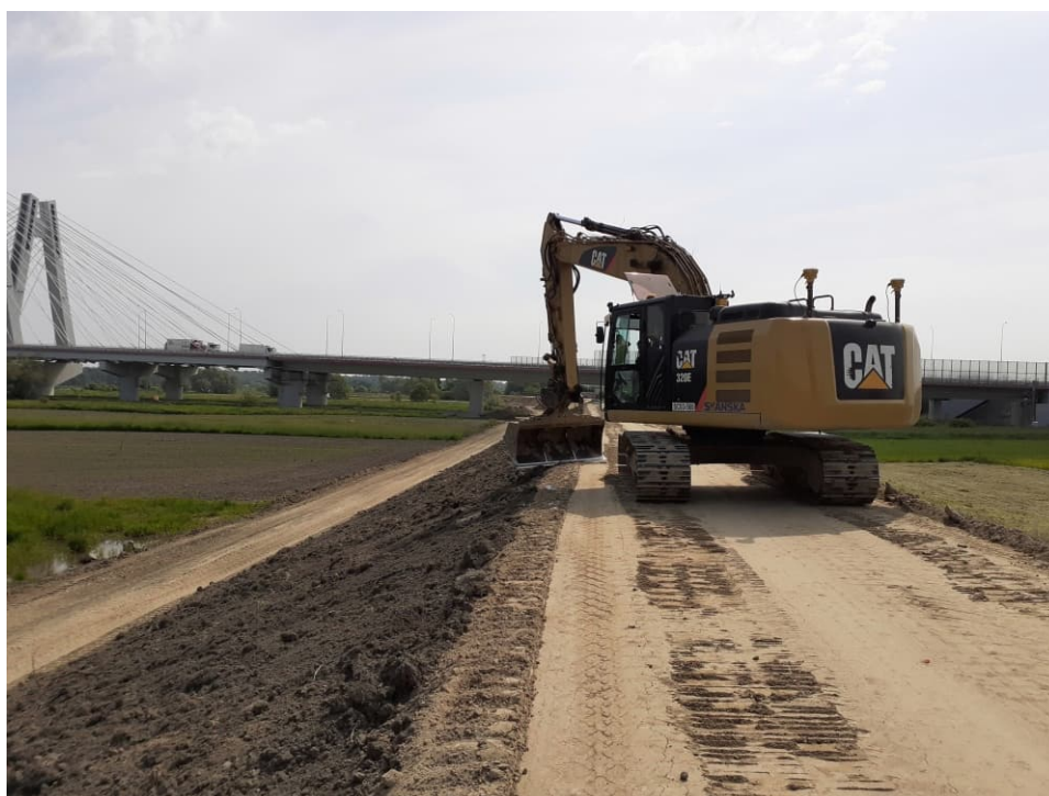
Fig. 52. Covering slopes of the flood embankment with a top-soil layer – the right Vistula embankment within Section 3.3 , status in the third decade of May 2023 (downstream view).
