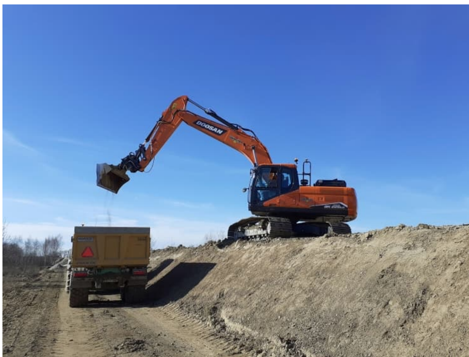
Fig. 47. Leveling the slopes of the flood embankment – the right Vistula embankment within Section 3.3 , status in the third decade of February 2022 (upstream view).
