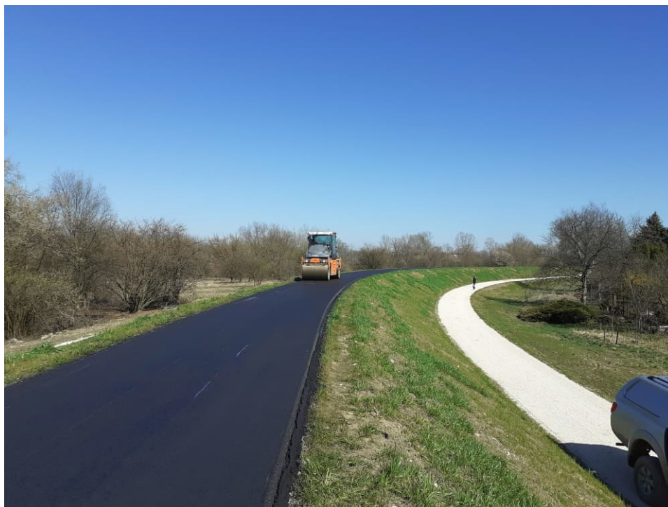
Fig. 54. Construction of a road on the crown of the flood embankment – the right Vistula embankment within Section 3.1 , status in the third decade of March 2023 (downstream view).
