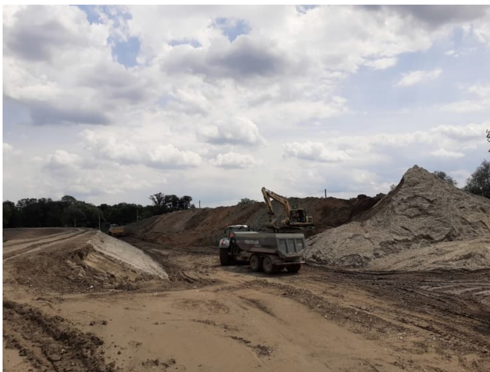
Fig. 43. Transport of earth masses for the reconstruction of a flood embankment – the right Vistula embankment within Section 3.2a , status in the first decade of July 2022 (downstream view).
