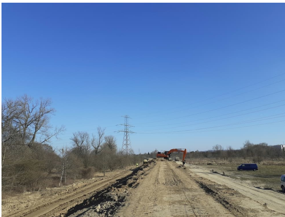
Fig. 45. Shaping the slopes of the flood embankment – the right Vistula embankment within Section 3.2a , status in the third decade of March 2022 (downstream view).
