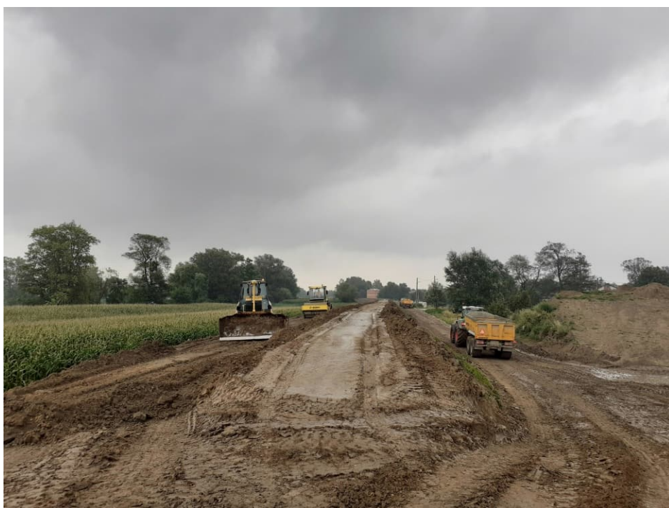
Fig. 44. Transport of earth masses for the reconstruction of a flood embankment – the right Vistula embankment within Section 3.2b , status in the third decade of July 2022 (downstream view).
