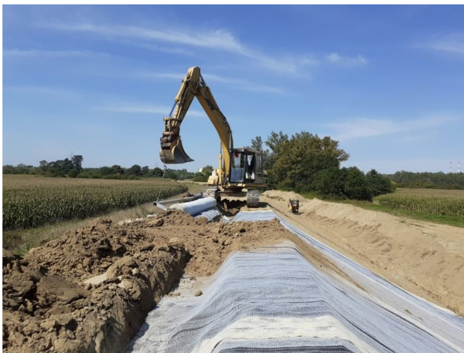
Fig. 49. Placement of bentomat on the slope of the flood embankment – the right Vistula embankment within Section 3.3 , status in the first decade of September 2022 (upstream view).
