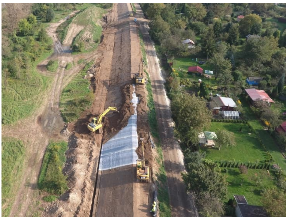
Fig. 50. Placement of bentomat on the slope of the flood embankment – the right Vistula embankment within Section 3.2a , status in the third decade of September 2021 (downstream view).
