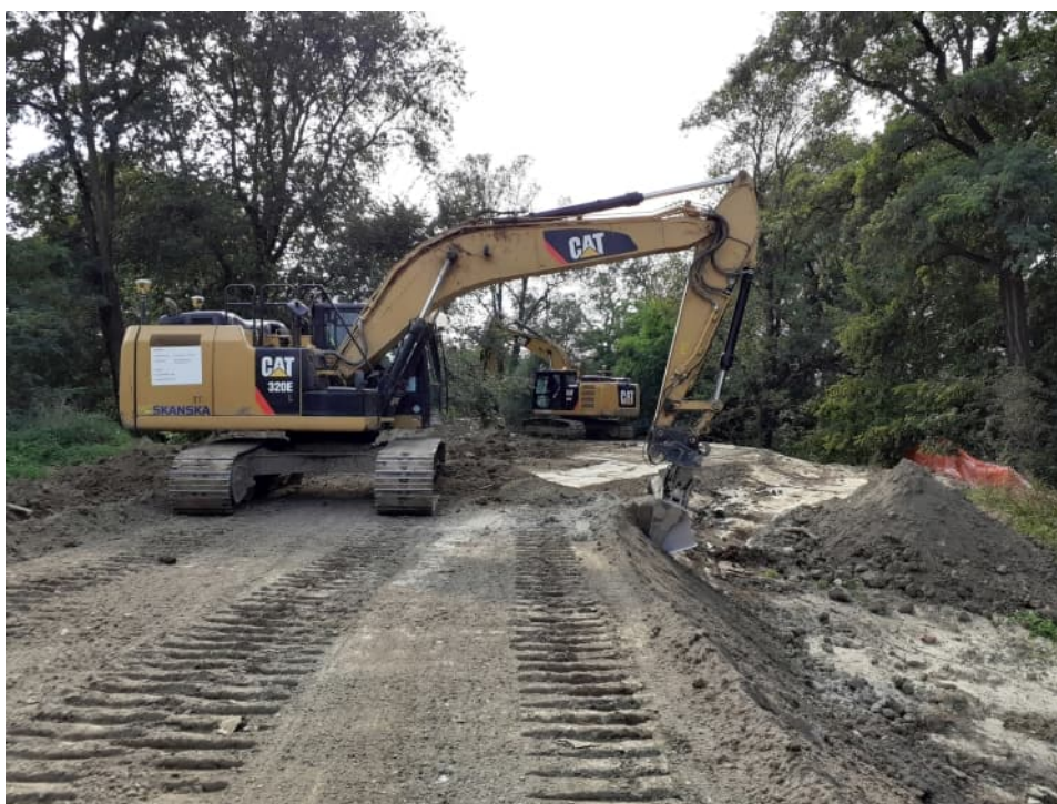
Fig. 46. Shaping the slopes of the flood embankment – the right Vistula embankment within Section 3.2a , status in the first decade of September 2022 (downstream view).
