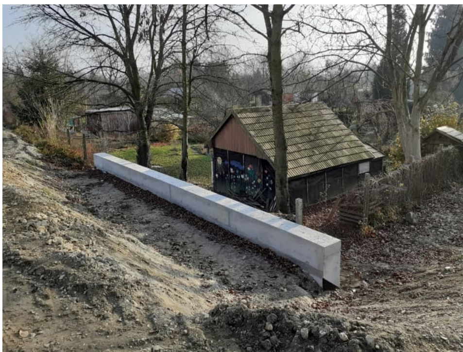
Fig. 39. Construction of a retaining wall – the right Vistula embankment within Section 3.2a , status in the second decade of November 2021 (downstream view).
