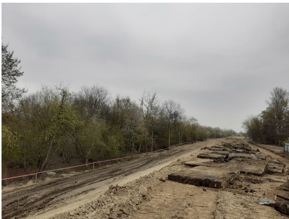
Fig. 21. Protection of trees and shrubs not intended to felling – the right Vistula embankment within Section 3.1 , status in the second decade of April 2022 (downstream view).
