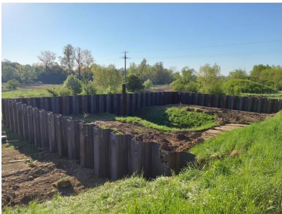
Fig. 36. A sheet piling protecting the embankment culvert during reconstruction – the right Vistula embankment within Section 3.4 , status in the second decade of May 2021 (downstream view).
