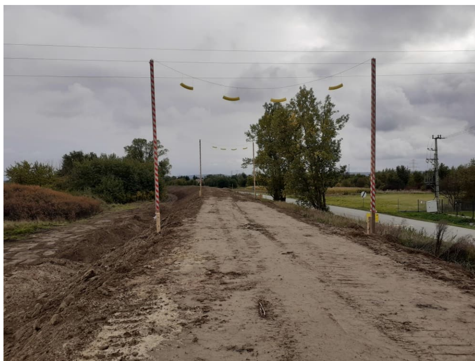
Fig. 18. Protection of hazardous sites under the power line – the right Vistula embankment within Section 3.4 , status in the third decade of September 2022 (downstream view).
