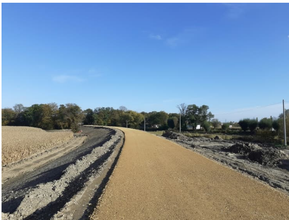
Fig. 53. Construction of a road on the crown of the flood embankment – the right Vistula embankment within Section 3.2a , status in the second decade of October 2022 (downstream view).
