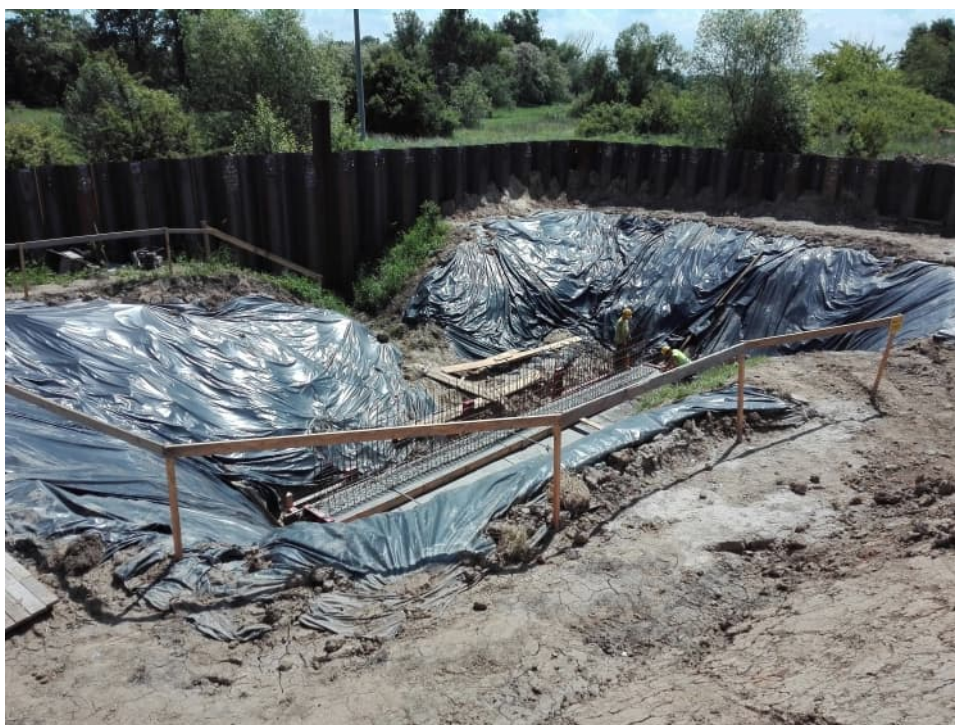
Fig. 37. Reconstruction of the embankment culvert – the right Vistula embankment within Section 3.4 , status in the third decade of May 2021 (downstream view).
