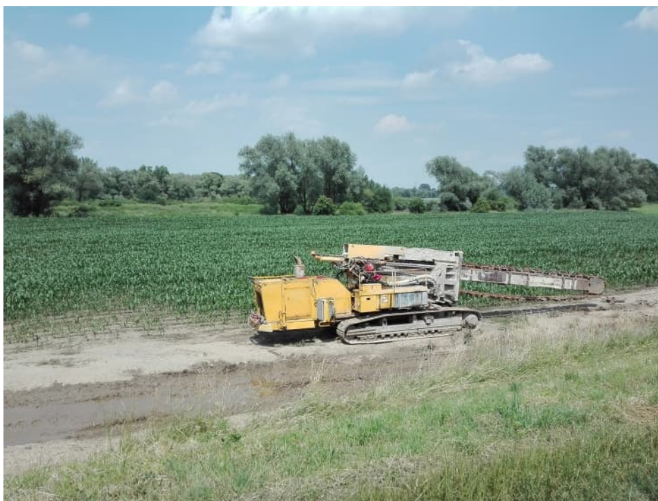
Fig. 33. Construction of a cement-bentonite barrier along the base of embankment – the right Vistula embankment within Section 3.2a , status in the third decade of June 2021 (downstream view).
