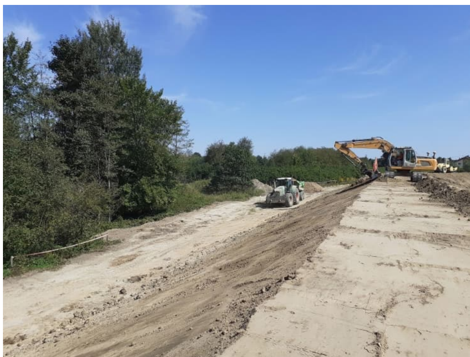
Fig. 48. Leveling the slopes of the flood embankment – the right Vistula embankment within Section 3.4 , status in the first decade of September 2022 (downstream view).
