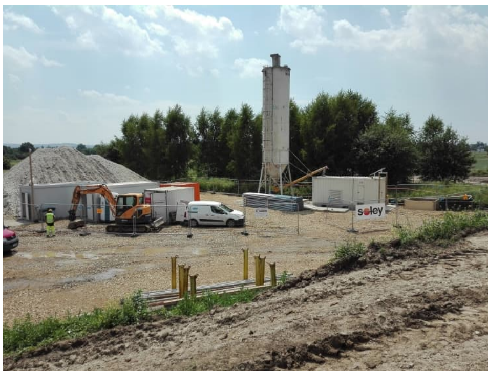
Fig. 34. Installation for producing a cement-bentonite mixture – the right bank of the Vistula within Section 3.3 , status in the third decade of June 2021 (upstream view).
