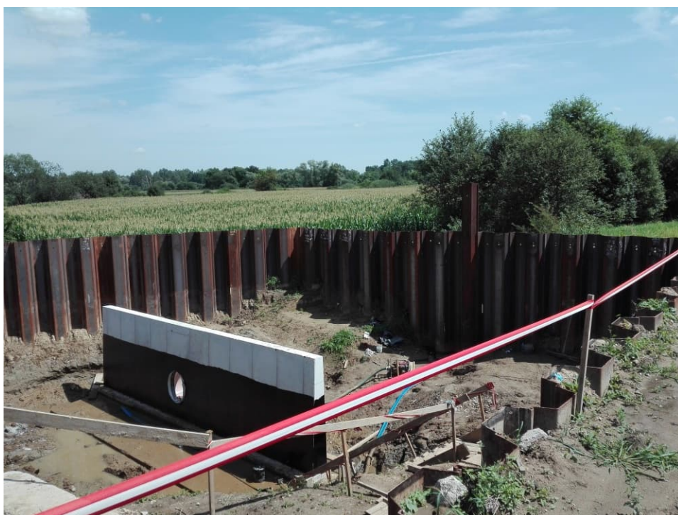
Fig. 38. Reconstruction of the embankment culvert – the right Vistula embankment within Section 3.4 , status in the third decade of July 2021 (upstream view).
