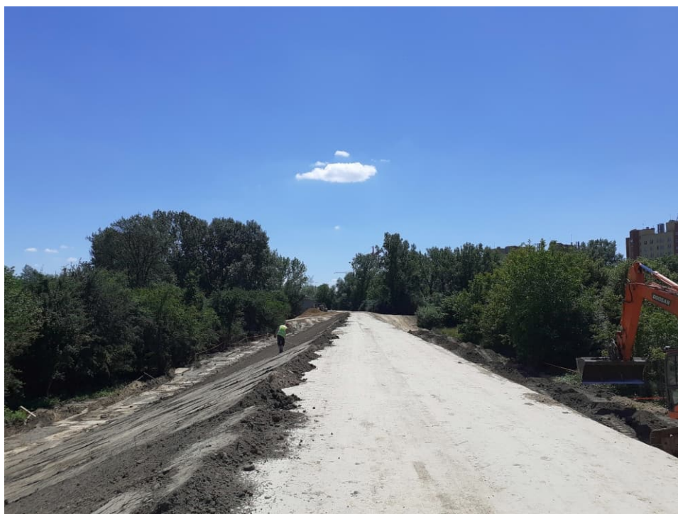
Fig. 51. Covering slopes of the flood embankment with a top-soil layer – the right Vistula embankment within Section 3.2a , status in the third decade of June 2022 (downstream view).
