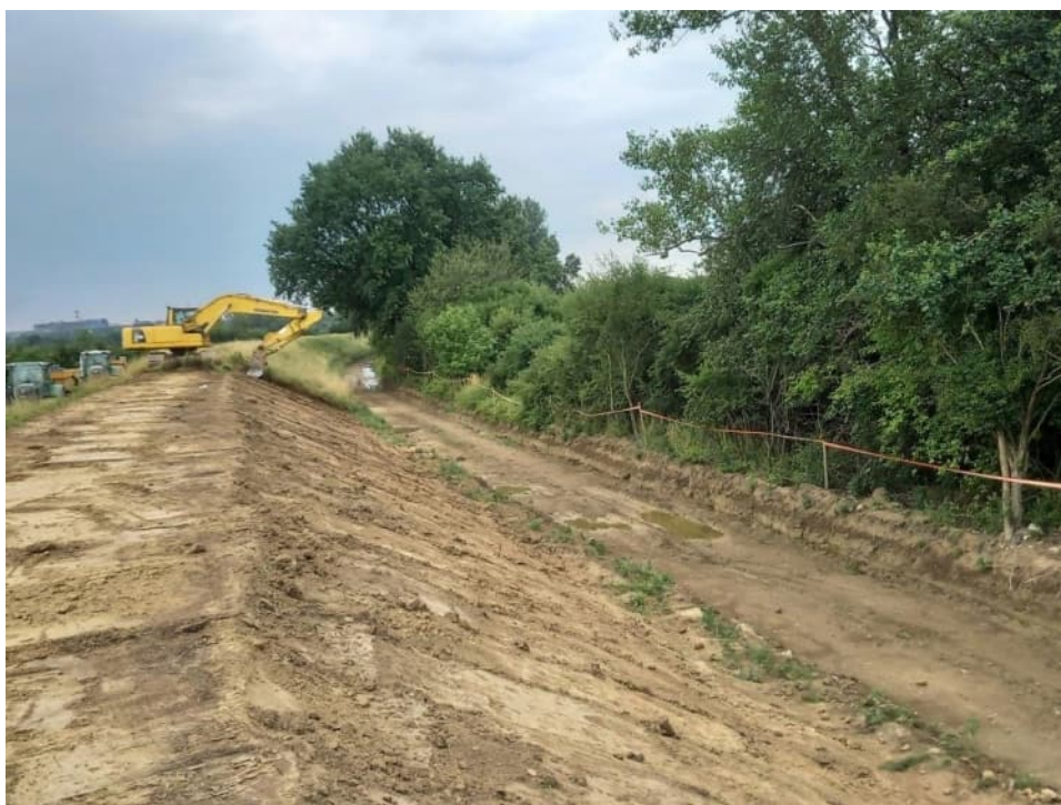
Fig. 29. Removal of a top soil layer – the right Vistula embankment within Section 3.4 , status in the first decade of July 2022 (upstream view).
