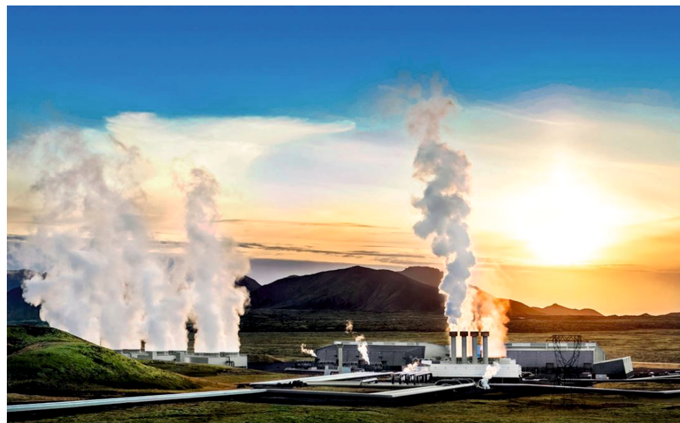
Geothermal plant, Hellisheiðarvirkjun (Iceland), source: Gunnar Svanberg
