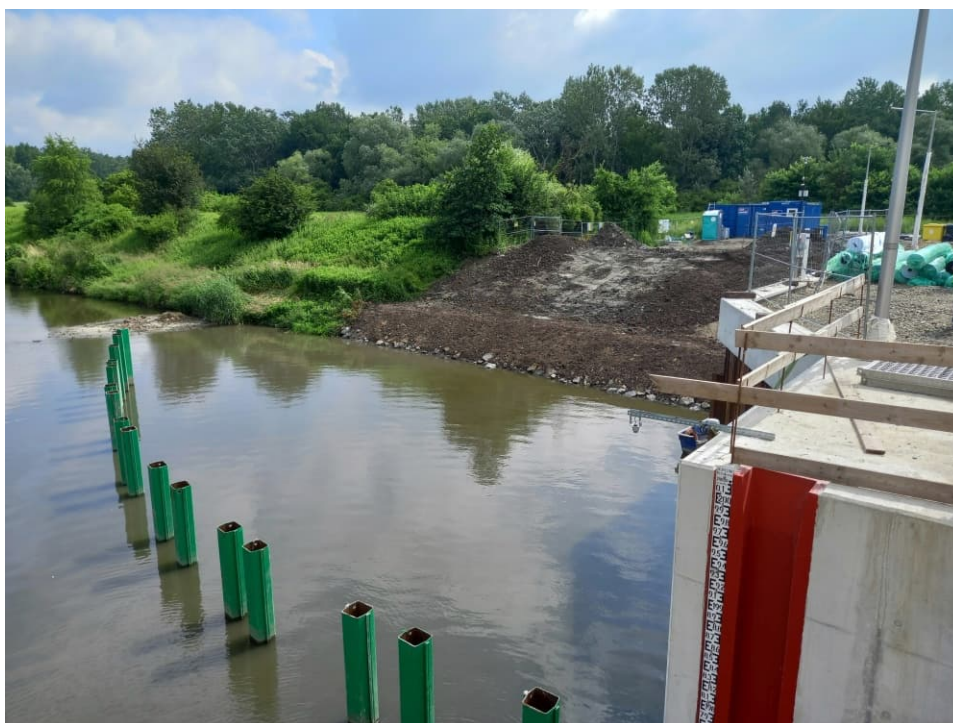
Fig. 44. Covering a bank slope with a top-soil layer on the eastern bank of the Kujawy port channel, status in the third decade of June 2023 (view towards the east).
