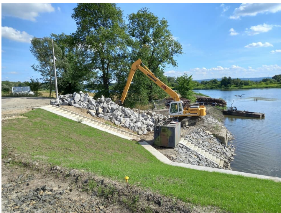
Fig. 42. A stone riprap for securing the bottom and slopes of the Kujawy port channel, status in the third decade of July 2023 (view towards the south).
