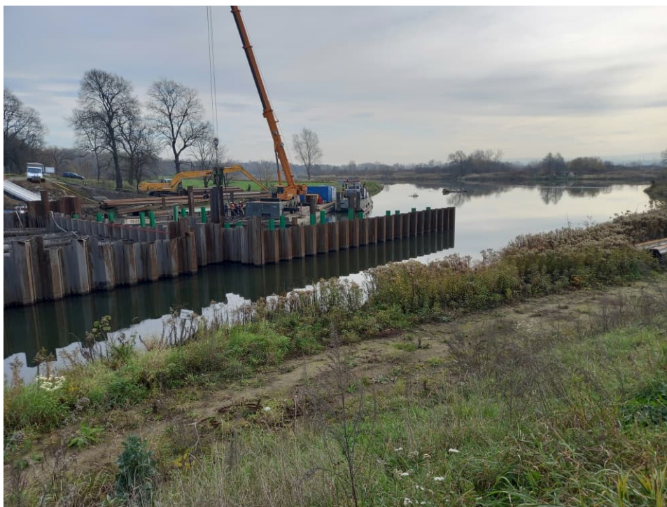
Fig. 27. Driving the sheet piles in the Kujawy port channel bed, status in the first decade of November 2022 (view towards the south).
