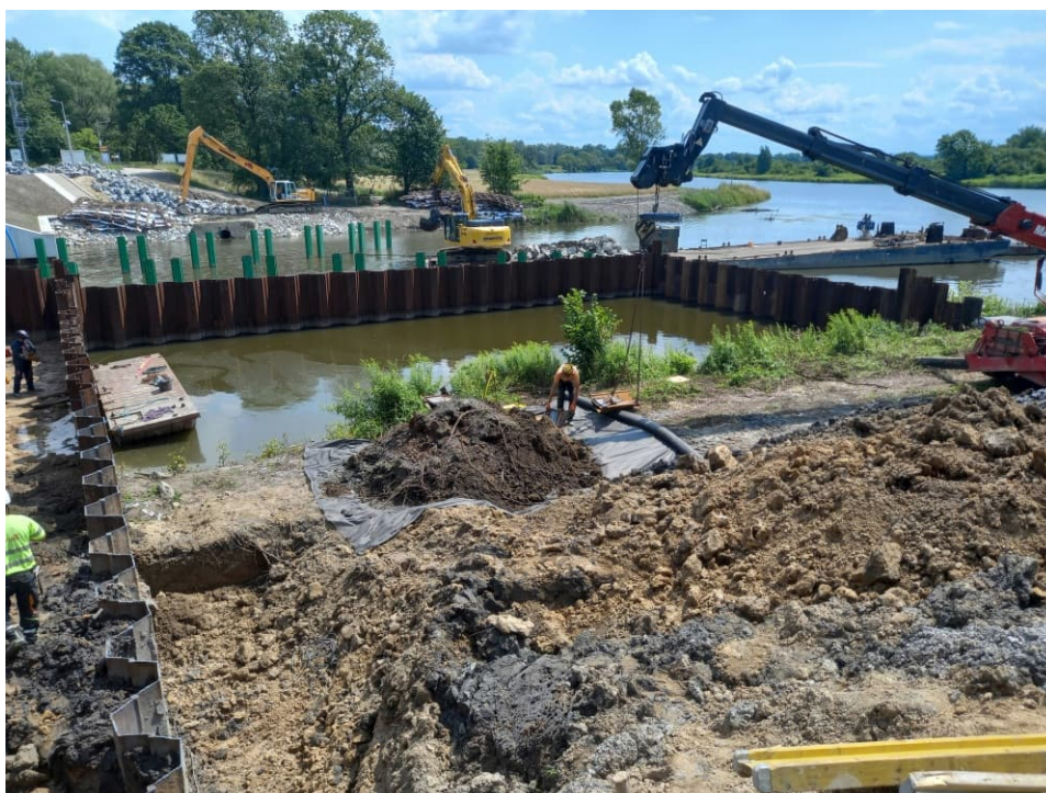
Fig. 22. Preventing the spread of foreign invasive plant species – protection of earth masses containing excavated knotweed roots, status in the second decade of July 2023 (view towards the east).
