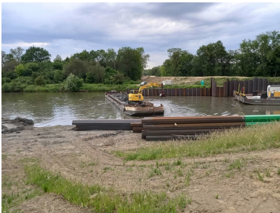
Fig. 25. Dredging of the Kujawy port channel bed south of the flood gate, status in the first decade of June 2022 (view towards the west).
