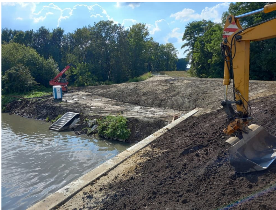
Fig. 43. Covering slopes of embankments with a top-soil layer on the western bank of the Kujawy port channel, status in the third decade of August 2023 (view towards the west).
