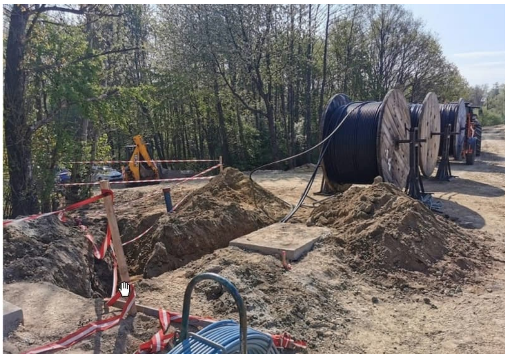
Fig. 23. Laying an electric cable to power the flood gate – works on the section along the left bank of the Vistula flood embankment, status in the first decade of May 2022 (view towards the east).
