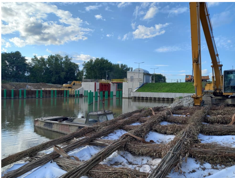
Fig. 41. A fascine mattress for securing the bottom and slopes of the Kujawy port channel, status in the first decade of August 2023 (view towards the north).
