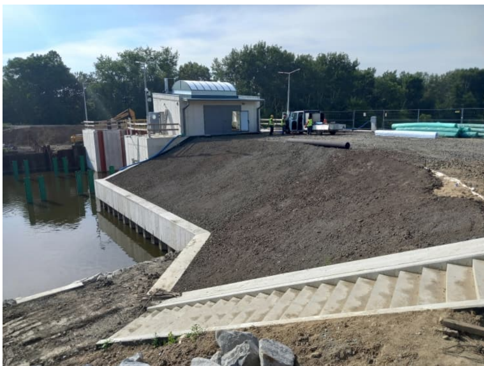
Fig. 34. Construction site of flood gate with a section of embankment connection on the eastern bank of the Kujawy port channel, status in the second decade of July 2023 (view towards the west).
