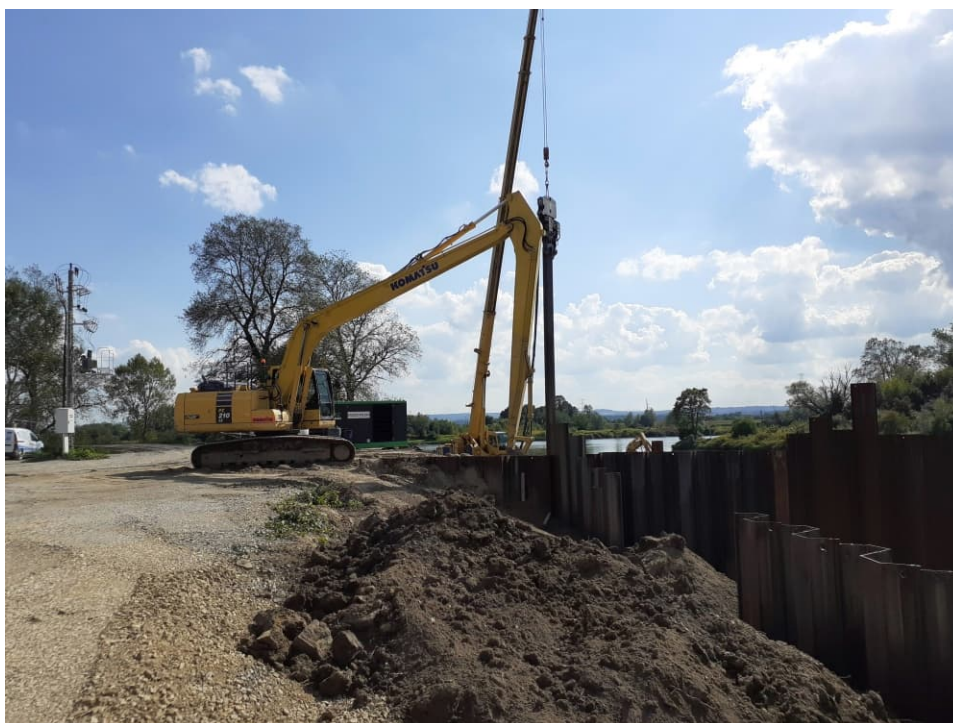
Fig. 28. Driving the sheet piles in the Kujawy port channel bed, status in the third decade of August 2022 (view towards the south).
