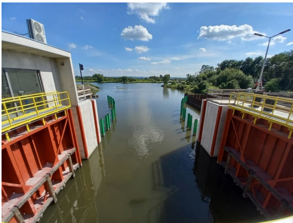
Fig. 39. The activated flood gate chamber in the Kujawy port channel, status in the third decade of July 2023 (view towards the south).
