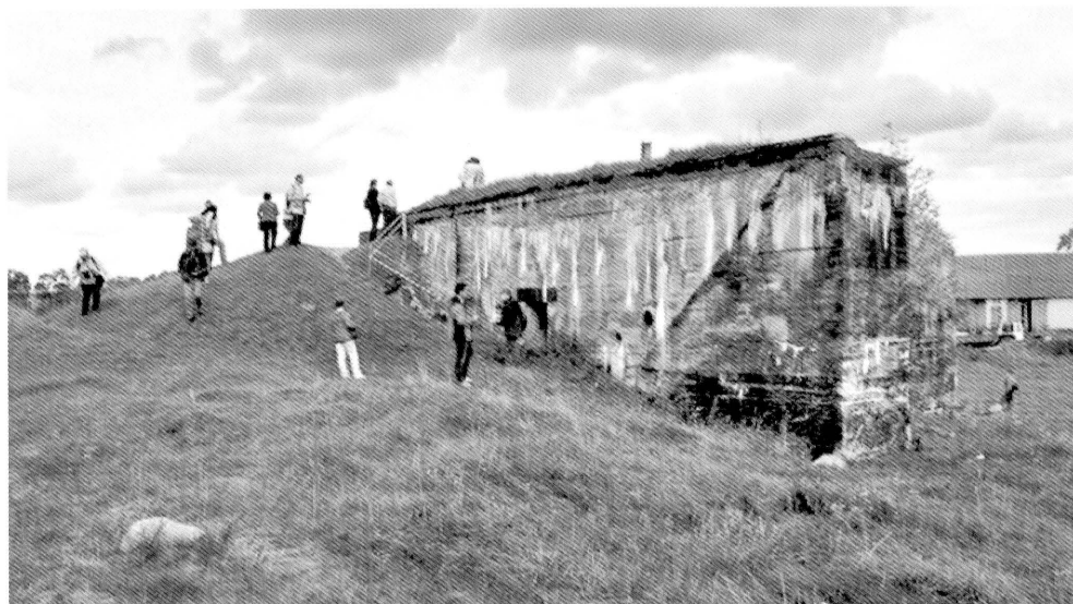
Catalogue bunker Regelbau 105c in Prawy Las. Tour of the frontier position as part of a session organised by the County Starosta's Office in Suwałki, 13 September 2009.
