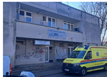
Façade of the Jesuit Refugee Service building
