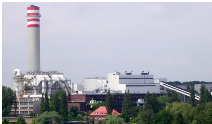
Fig. 3. Photo of EPS Pomorzany, gas humidification tower in front and EPS belonging to EB flue gas treatment plant in a photo centre. A scheme of installation for radiation flue gas purification at right (author's own work).
